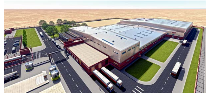
The new liquid detergent plant near Cairo in Egypt is designed as smart factory, where filling lines operate fully automated and are steered centrally to maximize resource efficiency, safety and quality. We have considered sustainability aspects right from the start when choosing the site location, during the construction phase up until the plant's official opening in mid-2017.
